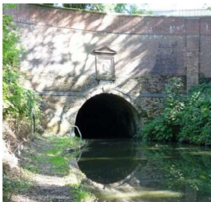
Brandwood Tunnel west portal
