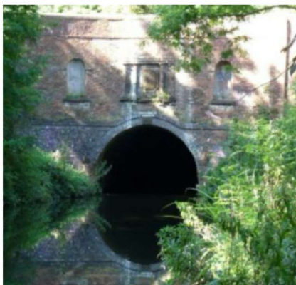
Brandwood Tunnel east portal
